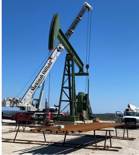
Figure 1: Pump installation at McLeod 1705
